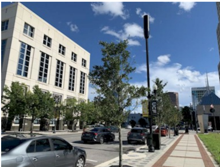
Photo: A small cell tower across the street from the Orange County Courthouse. The corresponding radio equipment is located in a portion of the adjacent
